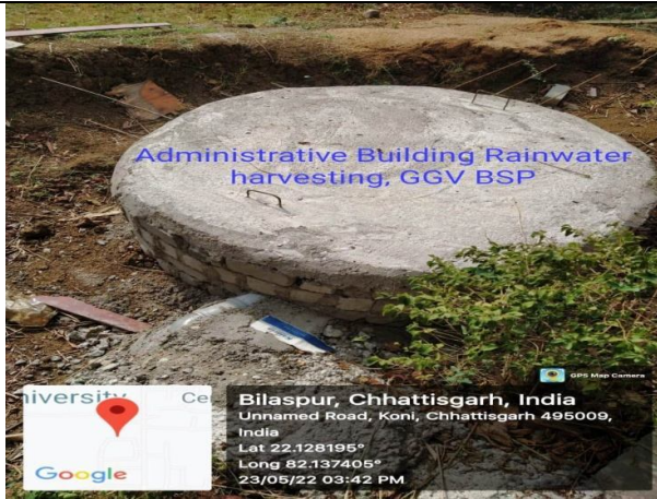
Rain Water Harvesting @ Administrative building
