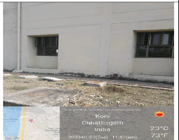
Rain Water Harvesting @ New Boys Hostel - B
