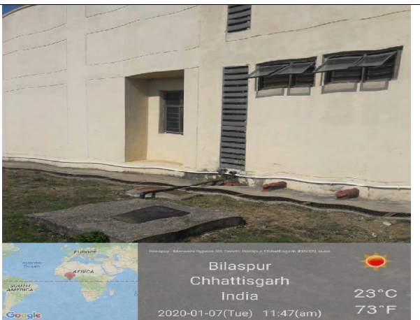
Rain Water Harvesting @ New Boys Hostel - A (Back Side)
